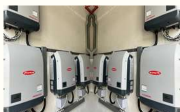
Figure 9: Inverter convert DC to AC
